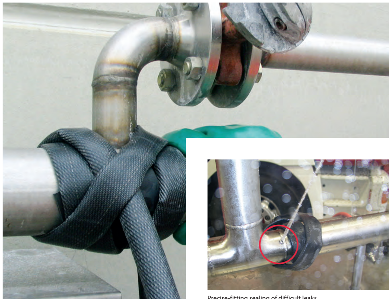
Precise-fitting sealing of difficult leaks
