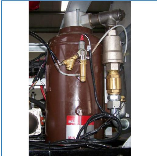
Separator tank for compressor oil
