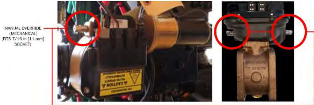
Figure 54. Mechanical Valve Override Shaft(s)
